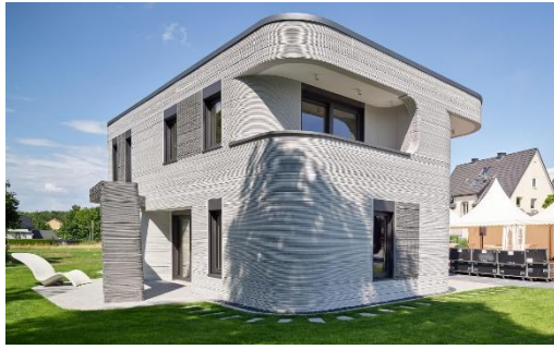
Figure 9 : Germany's first 3D-printed house From outside, the 3D-printed facade stands out with its rounded edges. Source: PERI
