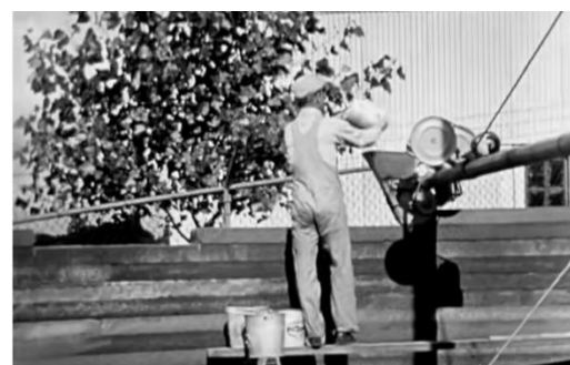
Figure 3 : A photo from short video Filmed in Valparaiso, Indiana in the late 1930's, William Urschel demonstrates his "Wall Building" machine in this video.
