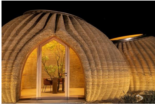
Figure 11: World's first 3D printed house made of local raw earth by Italian architecture studio Mario Cucinella Architects and Italy's pioneering specialists in 3D printing, Massa Lombarda, Italy
