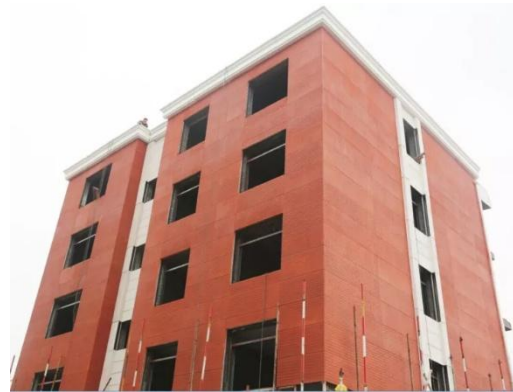
Figure 6 : The highest building ever constructed using 3D printing technology, Jiangsu province, China (Photo by: WinSun Decoration Design Engineering Co)
